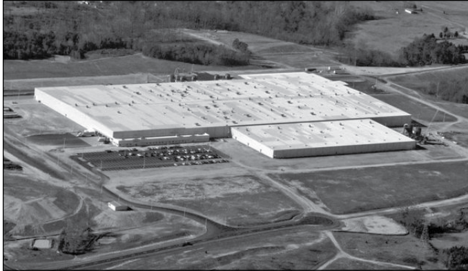
Swedwood Danville Virginia Plant
